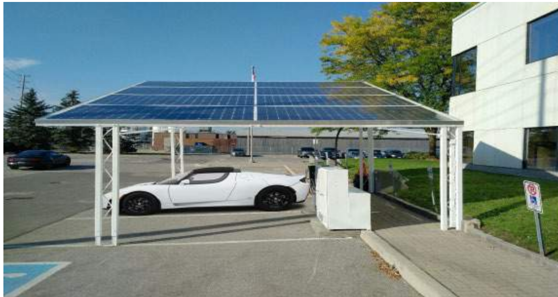
Notice the very light structure used to hold the panels
