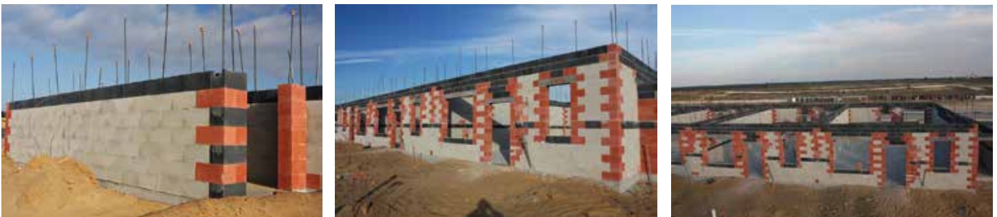
▼ Above – Cat5 Block homes under construction
